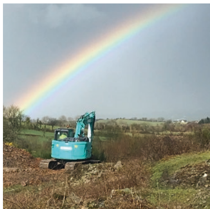
Trenching at Creenkill Gold Target
