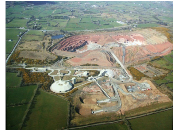
St. Gobain's Kingscourt open pit gypsum mine, County Monaghan
